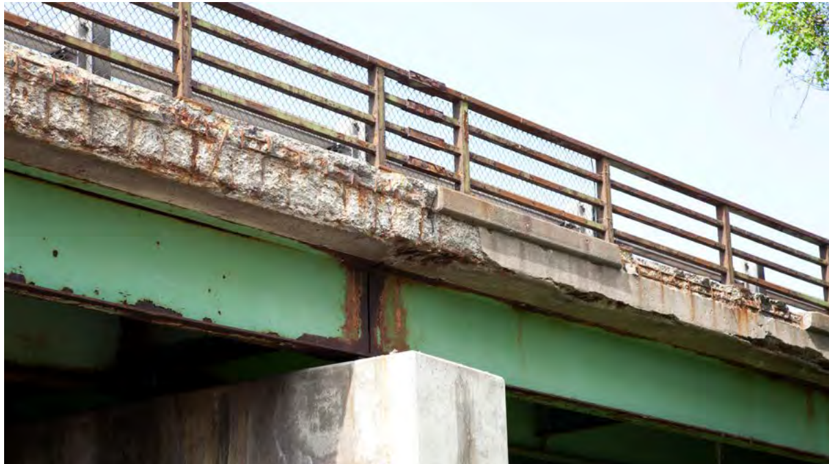
Carbonation on a highway bridge.
