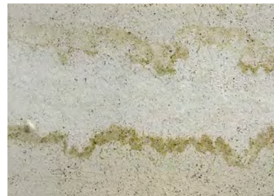
Old cementitious plaster stabilization (middle bright section). Salt decay and humidity attacks have been eliminated.
