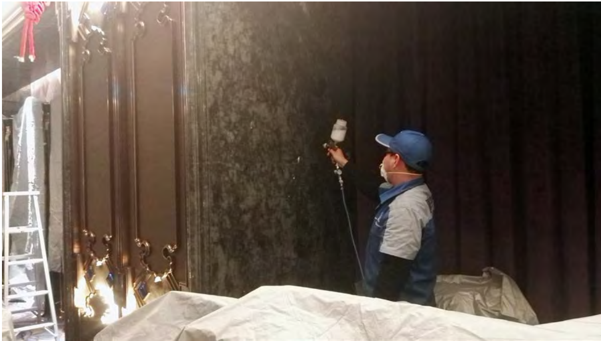
Application of SurfaShield T on vertical marble surface.
