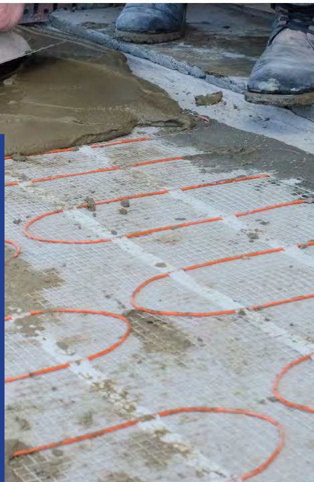
High thermal conductivity cement encasing of underground floor heating system, supported on FeatherPlast PT400.
