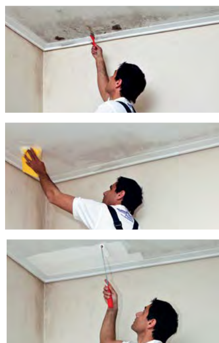
Mould removal and painting sequence by DeSalin AM and SurfaPaint AquaX.
