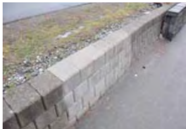
The effect of SurfaShield Cx in the fungi-rich environment of Norway, six months after installation.
