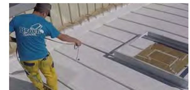
Application of SurfaPaint ThermoDry Elastomeric Roof on primed surface.
