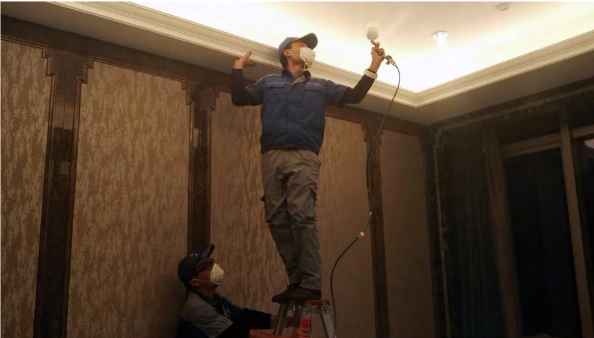
Application of SurfaShield C on painted ceiling.
