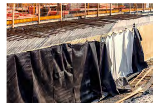
Basement Insulating system before landfilling.
