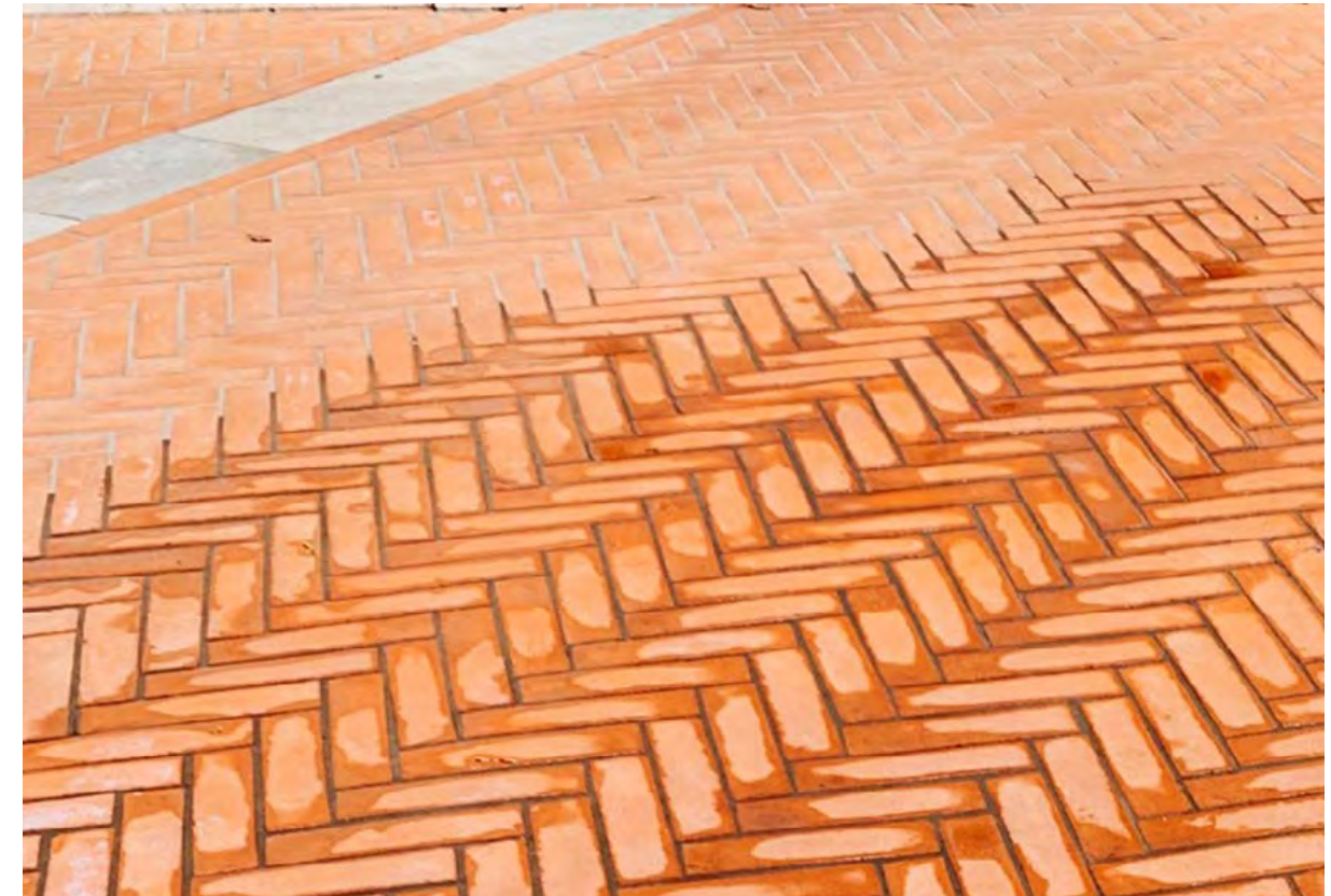
Freshly treated cotto floor tiles (bottom, right, wet) vis-a-vis untreated areas (top, left, dry). The final stage of treatment (SurfaPore C) has not concluded.
